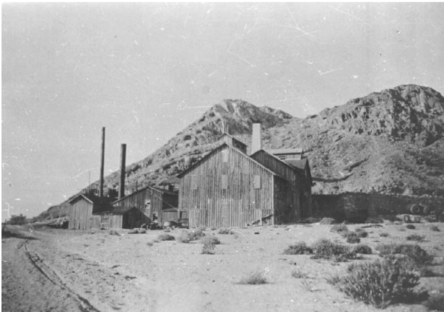
“One of the earliest innovations was the addition of steam-powered stamps. A forty-stamp mill was built by the Silver Peak and Red Mountain Gold and Silver Mining Company.” The mill was constructed in 1867. (Photograph courtesy of the Central Nevada Historical Society.)
